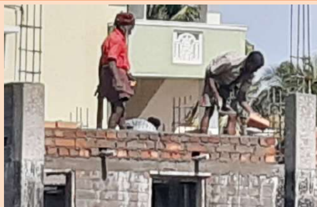
Mason packing bricks for constructing a wall between two pillars
